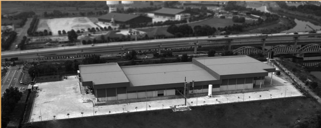
FFM Further Processing Plant, Pulau Indah, Klang.
